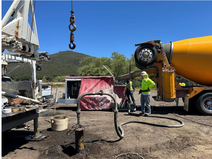
Installation of cement seal at Well No. 6.
