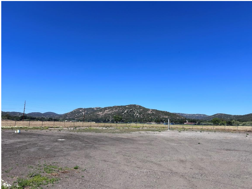
Site conditions as of June 9, 2026.
