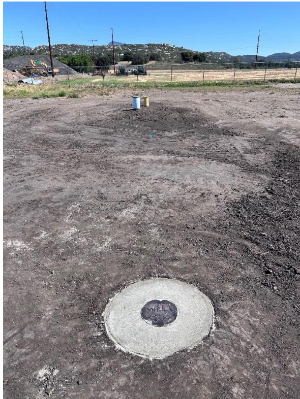
Site markers for the destroyed Well No. 6 and the capped discharge piping below ground.
