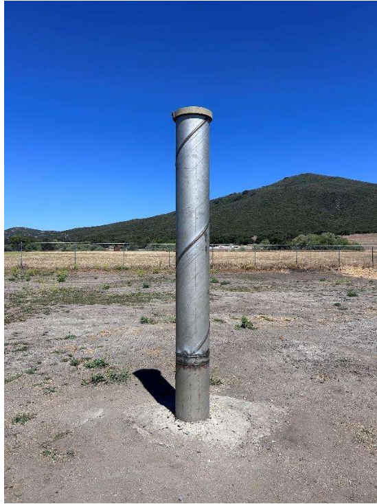
Completed Well No. 7.
