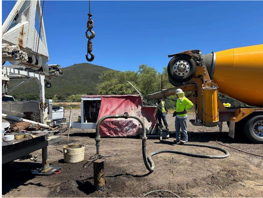
Installation of cement seal at Well No. 6.
